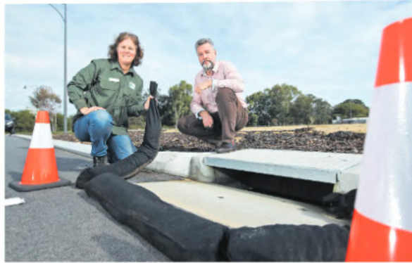
Perth NRM project officer Bronwyn Scallan and CEO Keith Pekin at one of the sites trialling silt control 'sausages'. Picture: David Baylis
