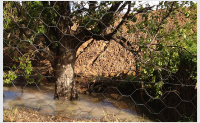
Example of inappropriate separation distances to vegetation and watercourses when infill is brought in
