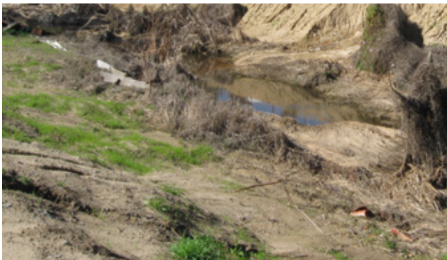
Historical example of a site subject to erosion without prevention measures to stop sediment entering a creek
