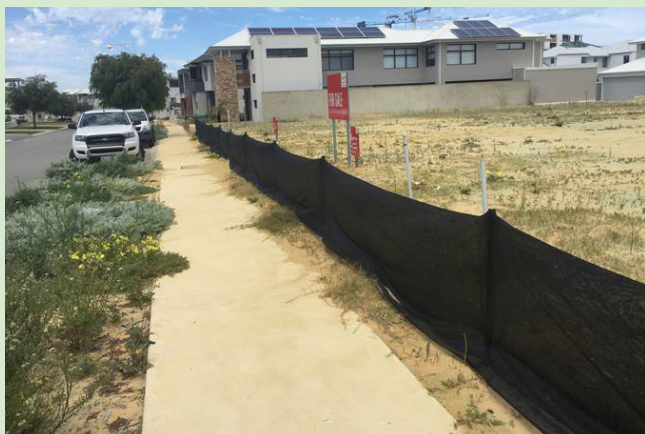
A marked decrease in sand leaving this block after a sediment control fence was installed.
