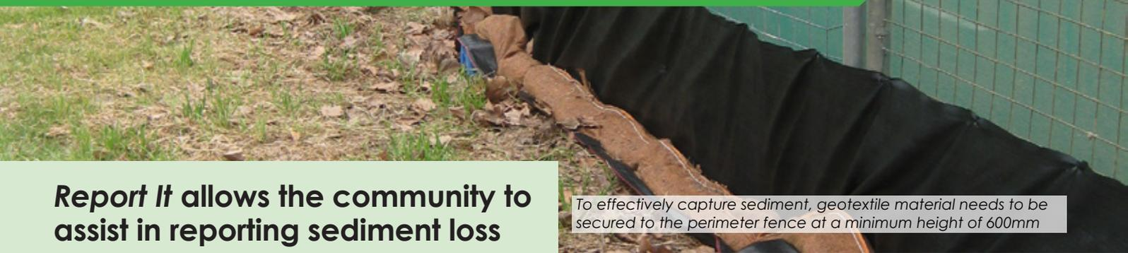
To effectively capture sediment, geotextile material needs to be secured to the perimeter fence at a minimum height of 600mm
