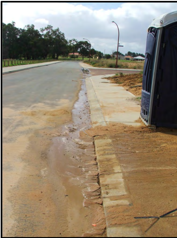
Figure 11: Erosion material transported to drains
